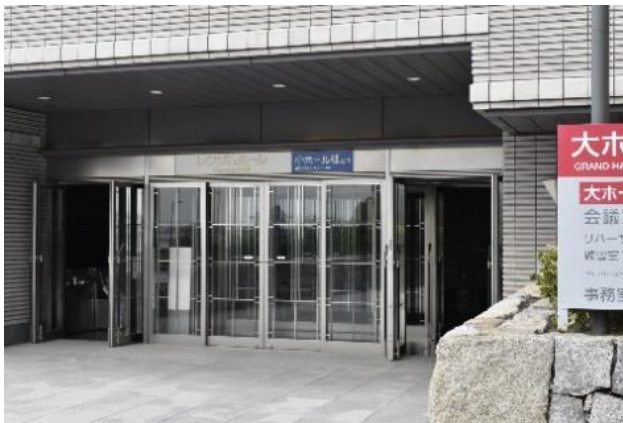
棟入口開放で換気
